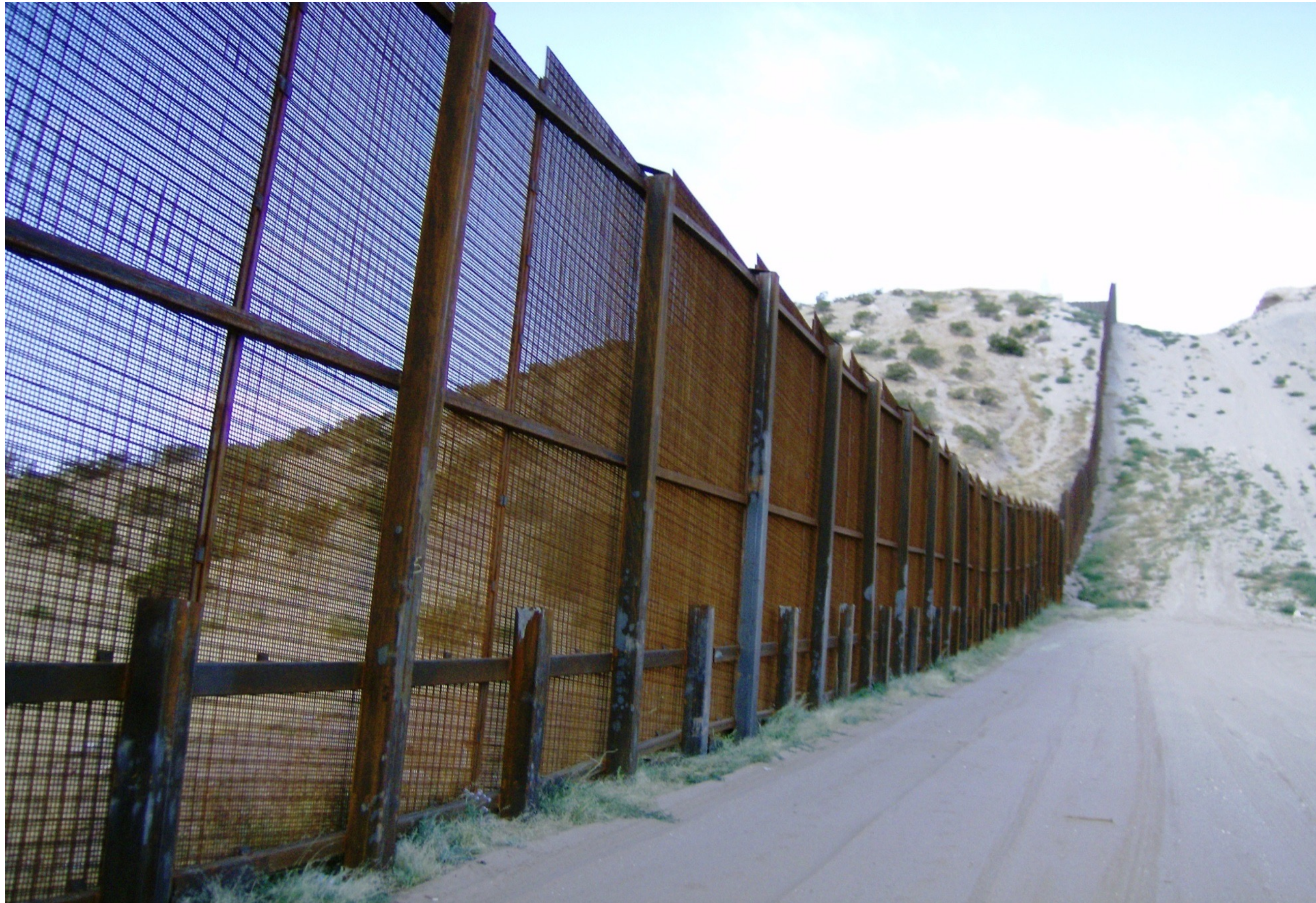
Strengthening the border fence
